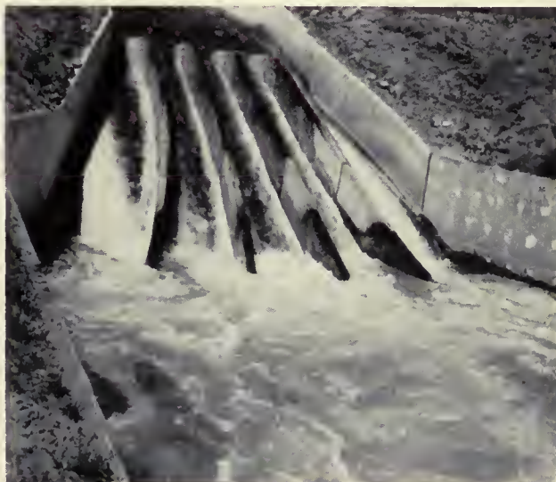
WHERE YOUNKIN DROWNED. —The upstream end of the stilling pool on the Riverton project in Wyoming into which Reuben Younkin was swept and drowned. Concrete baffles increased the hazard of turbulent water. Photo by S. T. Lorsen.
